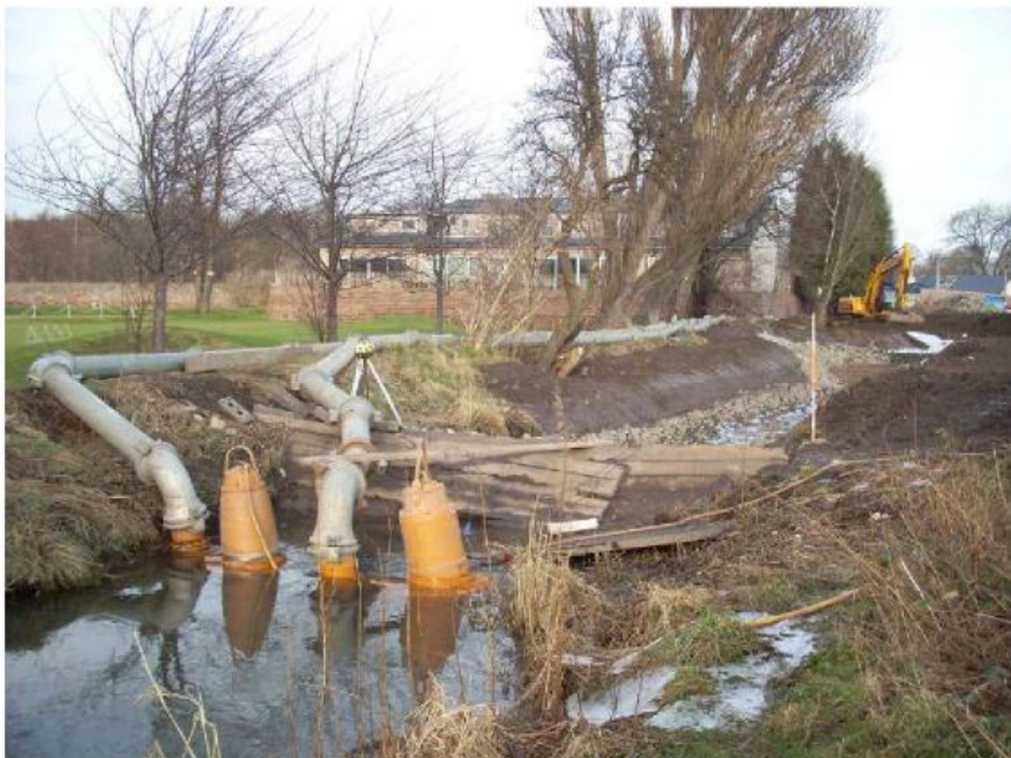
Plate 18: Watercourse Diversion (Full isolation – over pumping) 41
