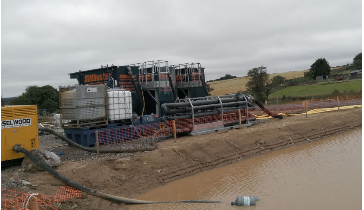
Plate 10: Settlement lagoon and Siltbuster pumping out water for treatment
