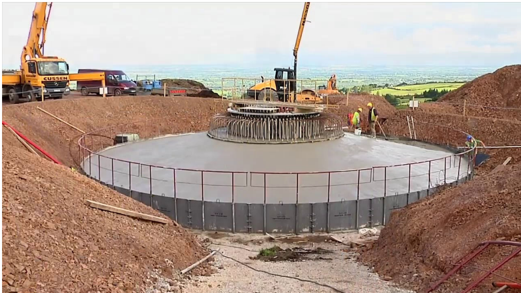
Plate 14: Shuttering for concrete foundation (wind turbine base)
